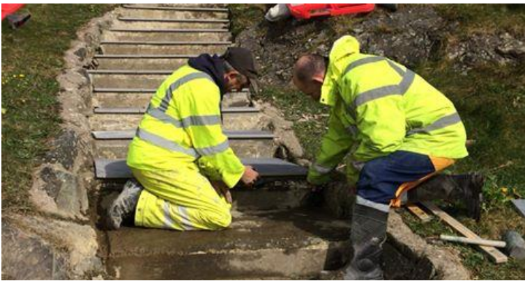
Pembrokeshire County Council's team installing the tiles.
